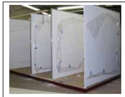
Fig. 4a Divider Walls Installed
