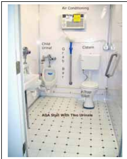
Fig. 15 ADA Unit Completed
