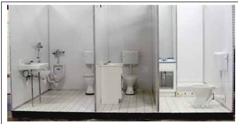
Fig. 11 Front View of Progress on 3 Stall Bldg.
