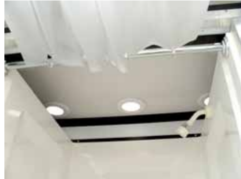
Rear Ceiling/Skylights Shower Head
