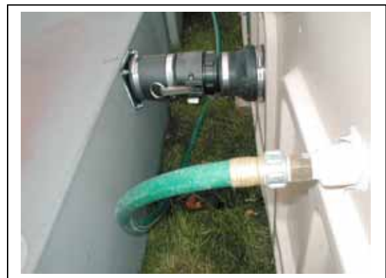
Water and Sewer Connection
