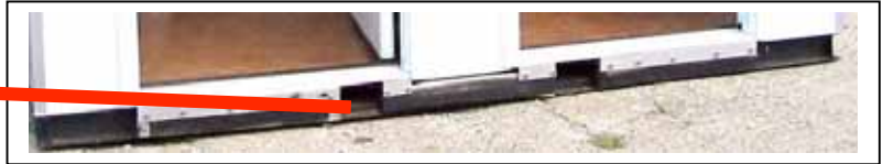
Fig. 2 Tine Ports (Steel Frame)
